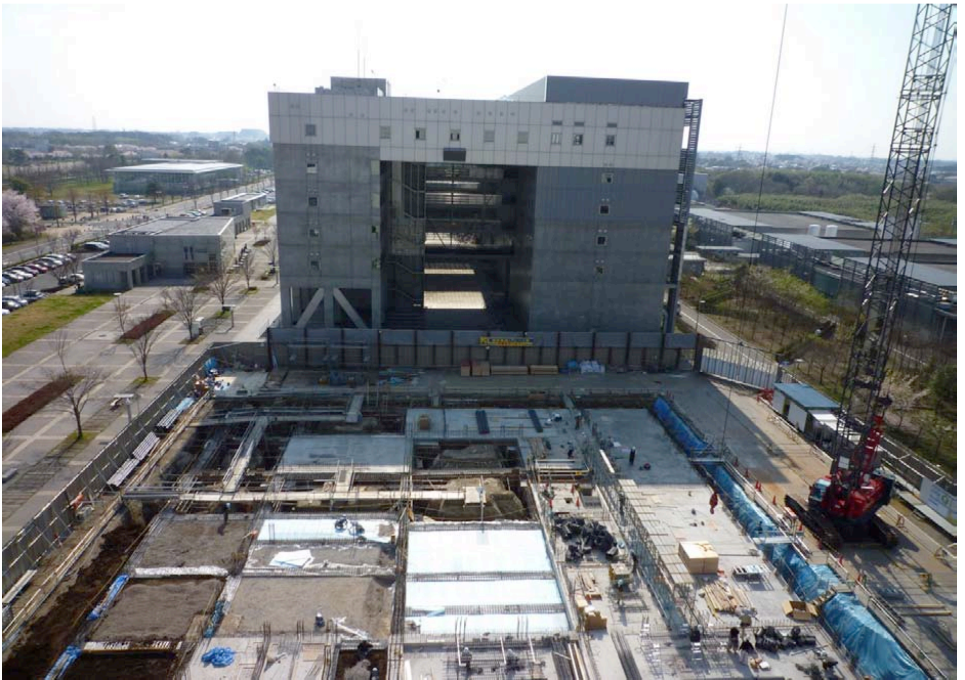
2009.02 IPMU New Building (Under construction)
