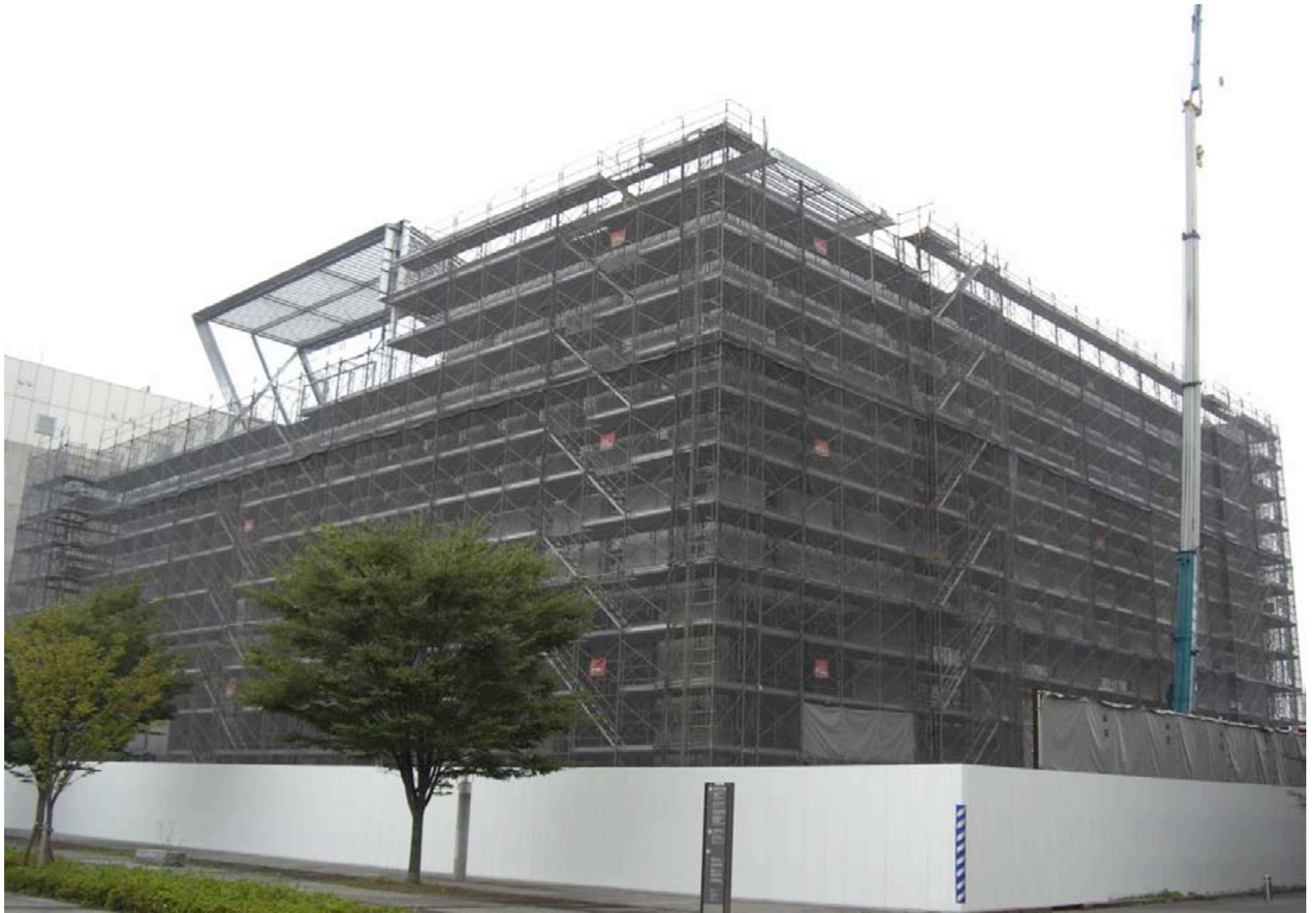
2009.10 IPMU New Building (Under construction)
