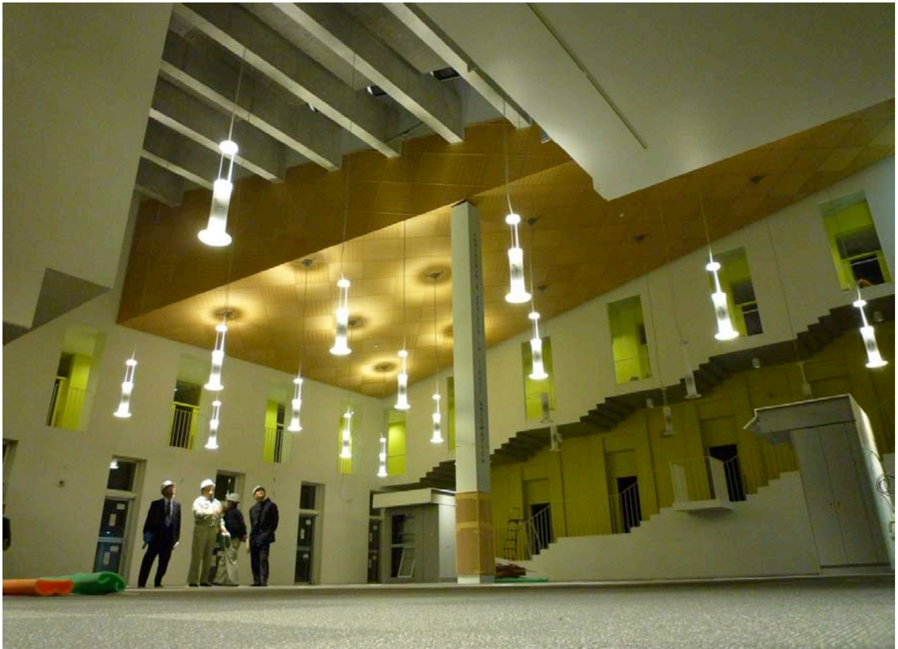
2009.12 IPMU New Building (Under construction)
