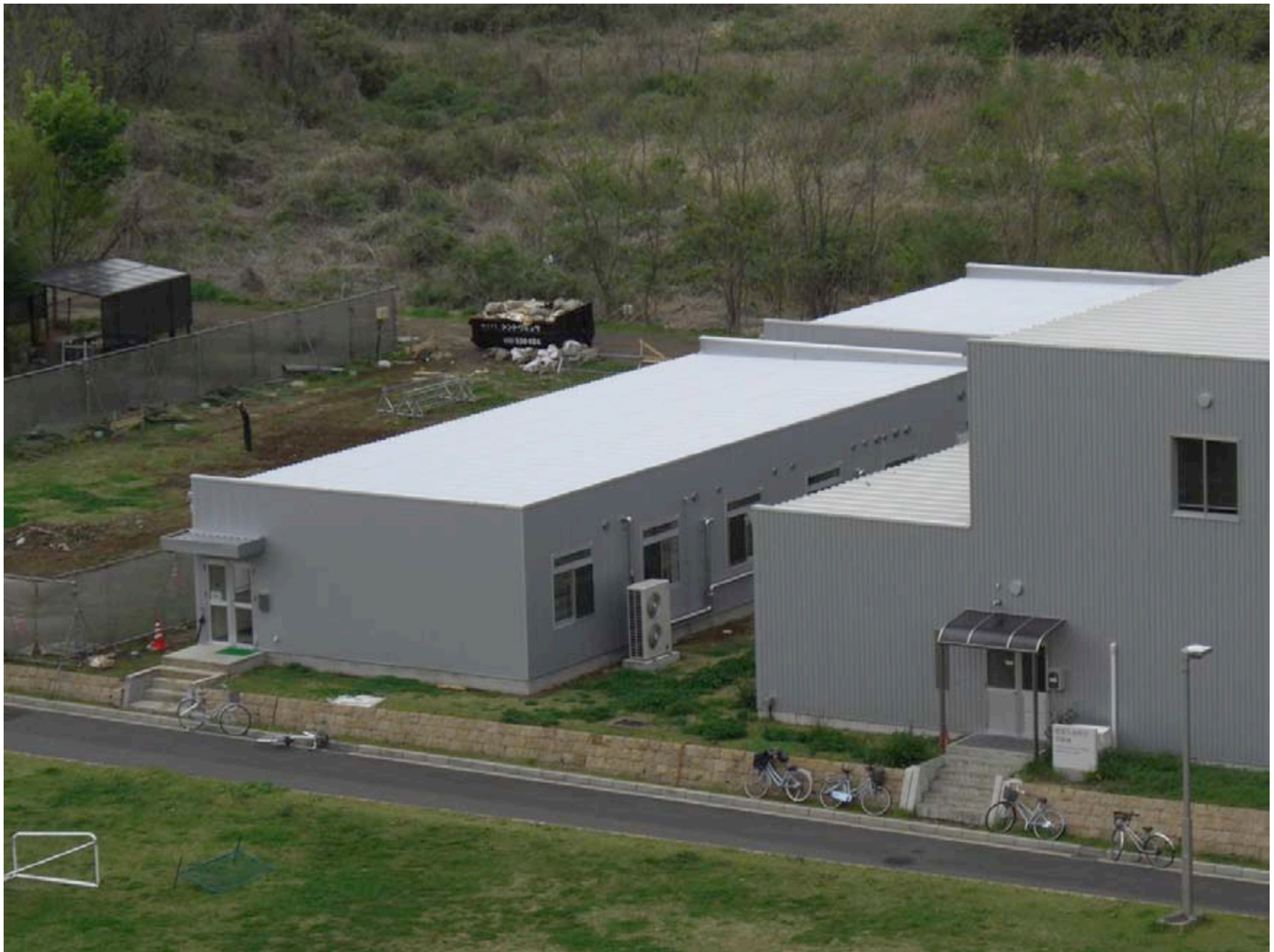
2008 IPMU prefab building
