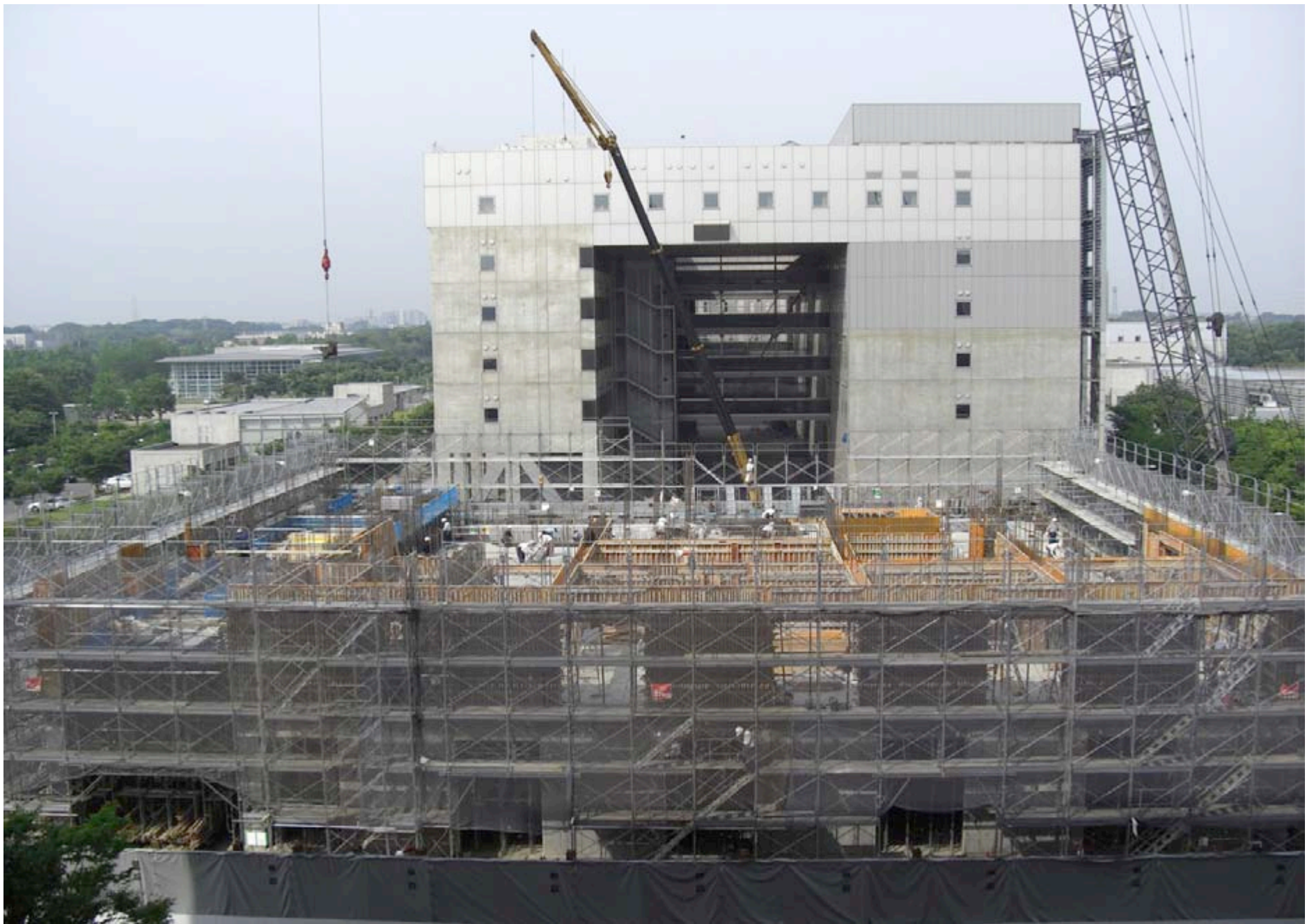
2009.05 IPMU New Building (Under construction)
